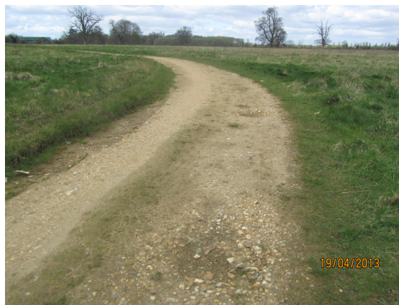
Surface in disrepair across North Field due to no maintenance and vehicular damage
