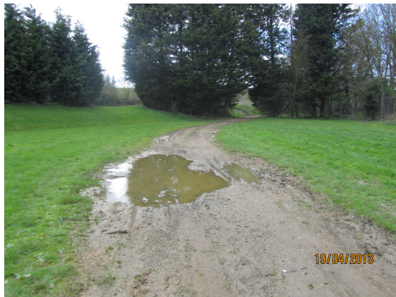
Drainage problem on southern end of path leading to Major's Farm Road gate
