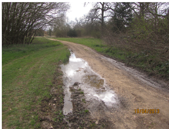
Surface in disrepair across North Field due to no maintenance and vehicular damage
